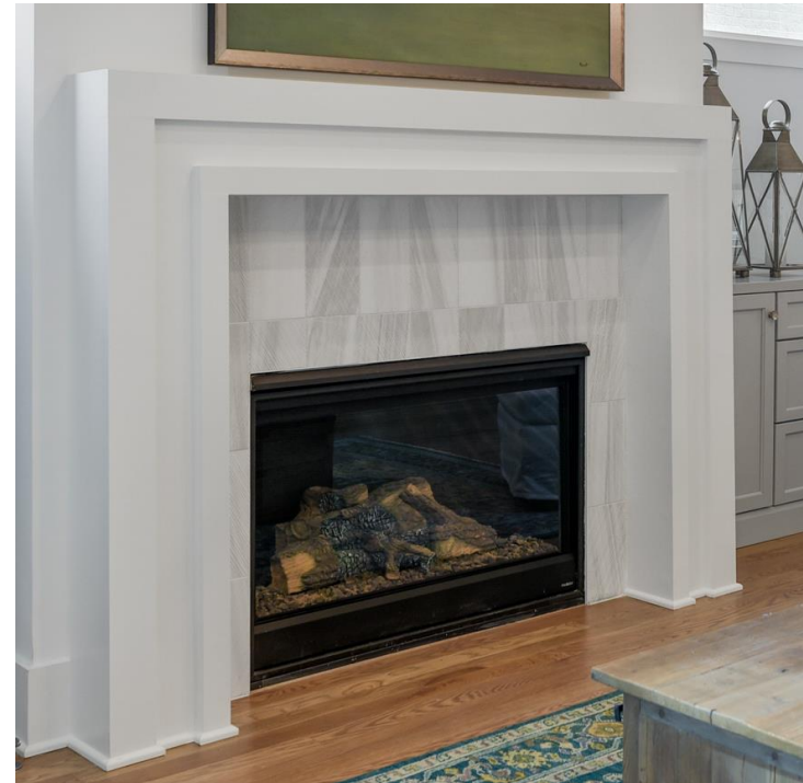
TRIM BUILT WOOD MANTLE STYLE #2, PAINTED THE TRIM COLOR NO HEARTH – HARDWOOD TO RUN TO FIREPLACE CHASE
